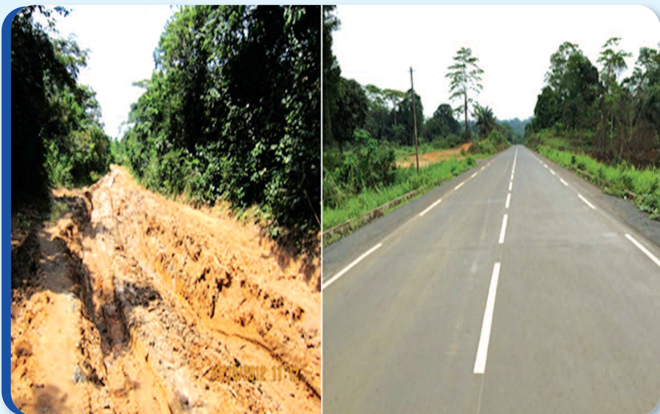
The Mamfe - Ekok road before and after construction.
