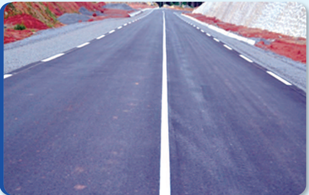
The newly constructed section of the ring road from Ndop to Kumbo.
